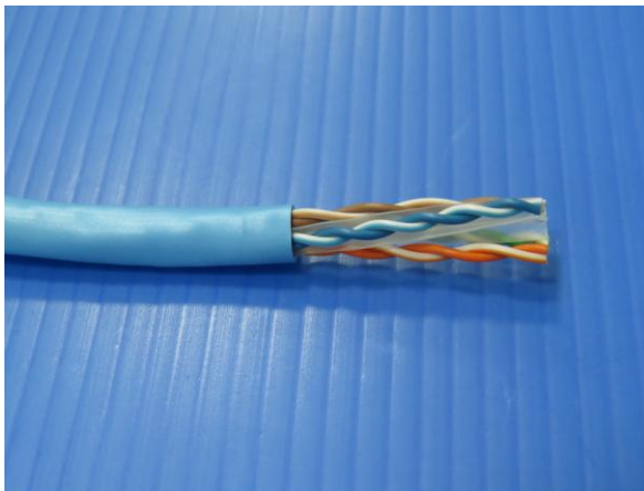
2. Strip and removed 20mm of jacket.
